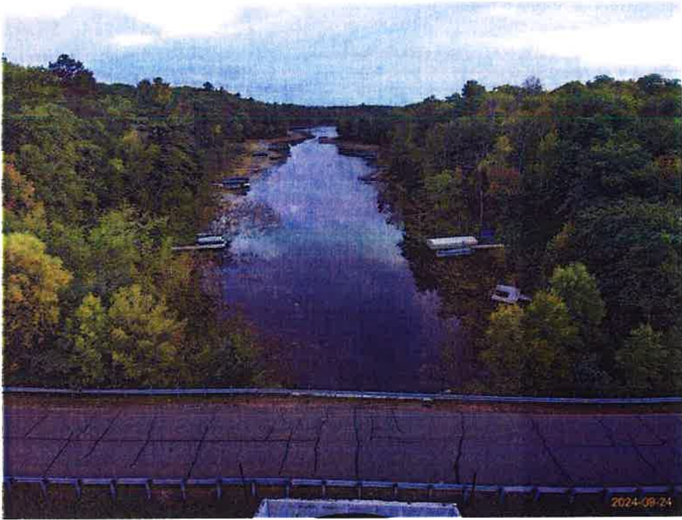
Photo 3 - NORTH CHANNEL LOOKING NORTH
