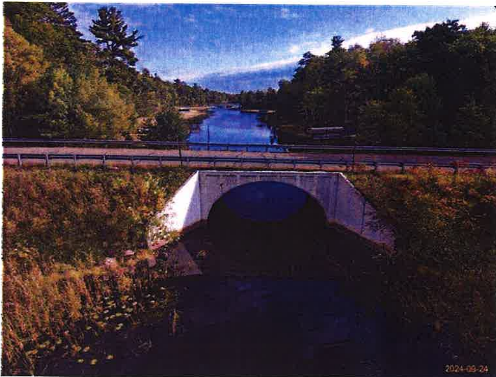
Photo 2 - SOUTH PROFILE LOOKING NORTH
