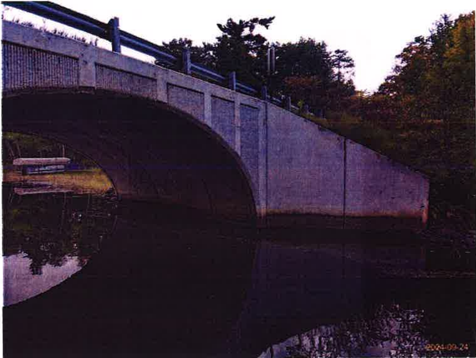
Photo 8 - EAST CULVERT WALL LOOKING NORTHEAST
