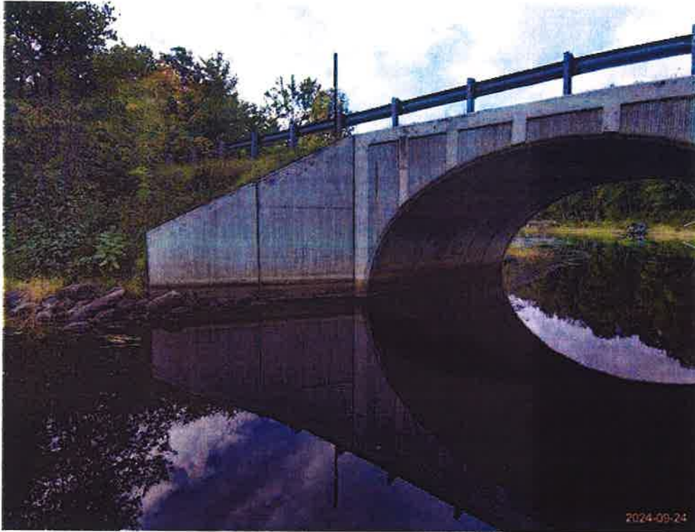
Photo 9 - EAST CULVERT WALL LOOKING SOUTHEAST
