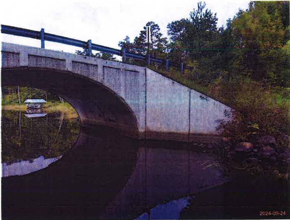
Photo 7 - WEST CULVERT WALL LOOKING SOUTHWEST
