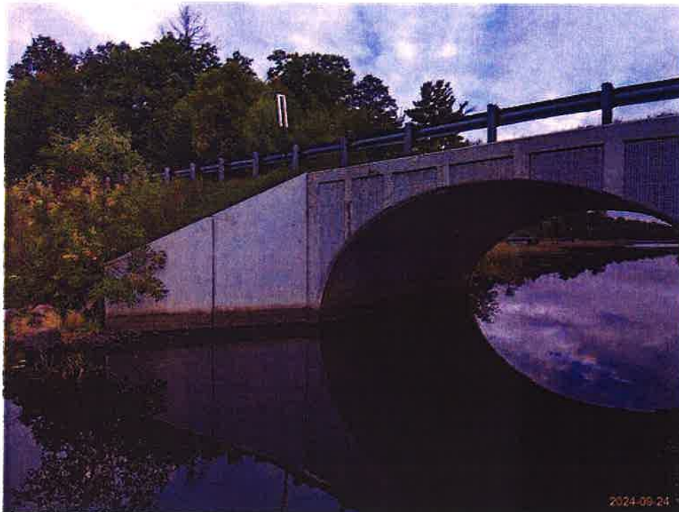
Photo 6 - WEST CULVERT WALL LOOKING NORTHWEST
